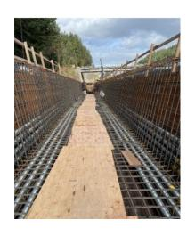
Rebar placed for I-5 overcrossing stem walls
