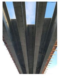
Guideway precast panels placed between girders
