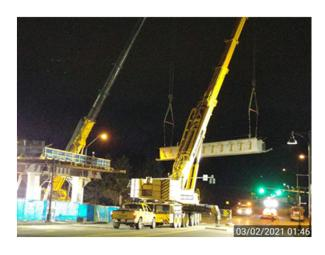
Girder installation over 236<sup>th</sup> St SW, east of I-5 at Mountlake Terrace Station
