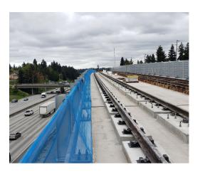
Elevated guideway direct fixation track installation in North Seattle
