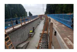
Cast-in-place tub girder concrete at I-5 overcrossing
