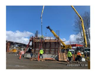
Placing shear wall concrete at the Lynnwood Station Garage
