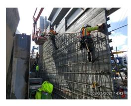
Rebar placement for cast-inplace concrete wall fascia in Lynnwood
